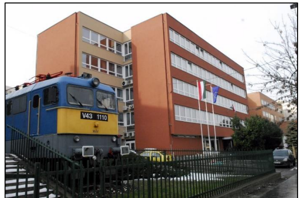
BC - Bécsi út 94., District III. Kálmán Kandó Faculty of Electrical Engineering – KVK, Mobility Department
